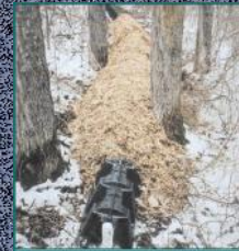
Infiltrator chamber replaces rock in at-grade (Picture not taken in Iowa!)
